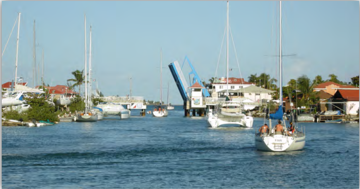
SANDY GROUND BRIDGE~FRENCH SIDE: THE OPENING IS 32ft WIDE BUT THE DEPTH IS LIMITED
